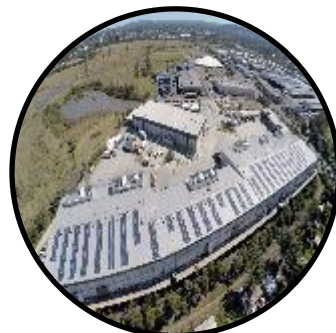
Commercial and Industrial Rooftop
